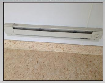
**BASEBOARD HEATING SYSTEM -** A must for the year-round roving workshop. The self-contained unit comes with an optional adjustable thermostat control or wall-mount thermostat.
